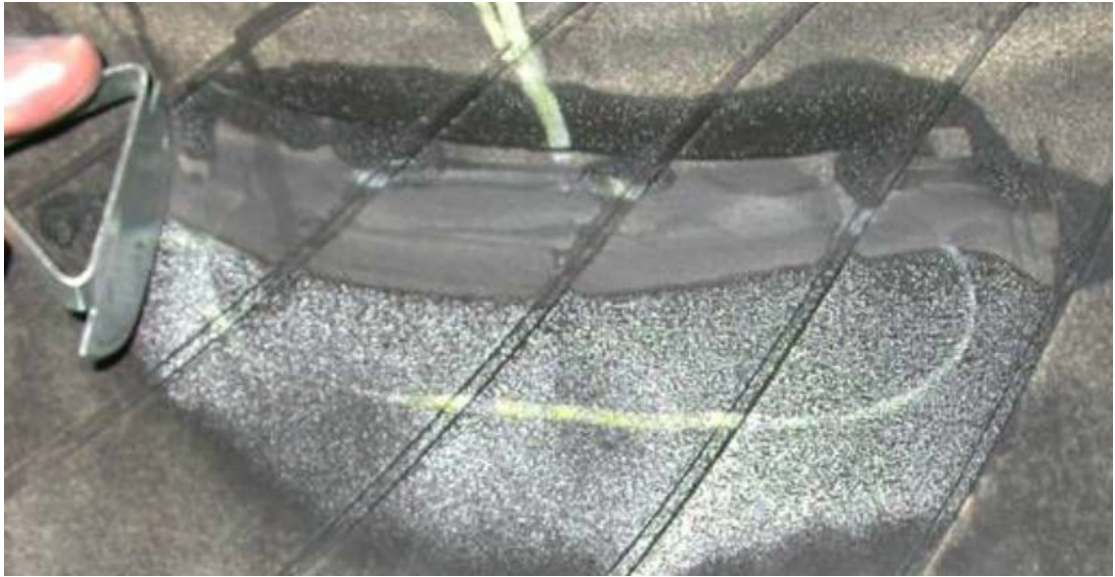
Using a scraper to remove contaminants on the surface
